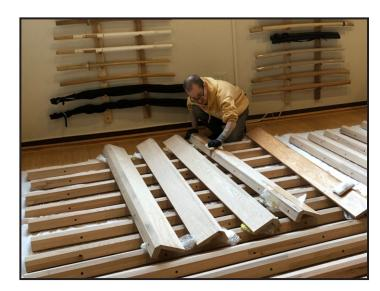
The second delivery of materials was made on Friday, February 24, and consisted of the subfloor components. Assembled, the subfloor is two layers of ½-inch birch plywood. The bottom layer comes with six-inch, steel springs attached—pieces to be placed on the outside edges of the subfloor have double the number of springs along the edge(s). In total, our system has almost 1,500 springs.
